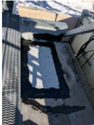
Temporary repair until roof can be replaced in warmer conditions.
